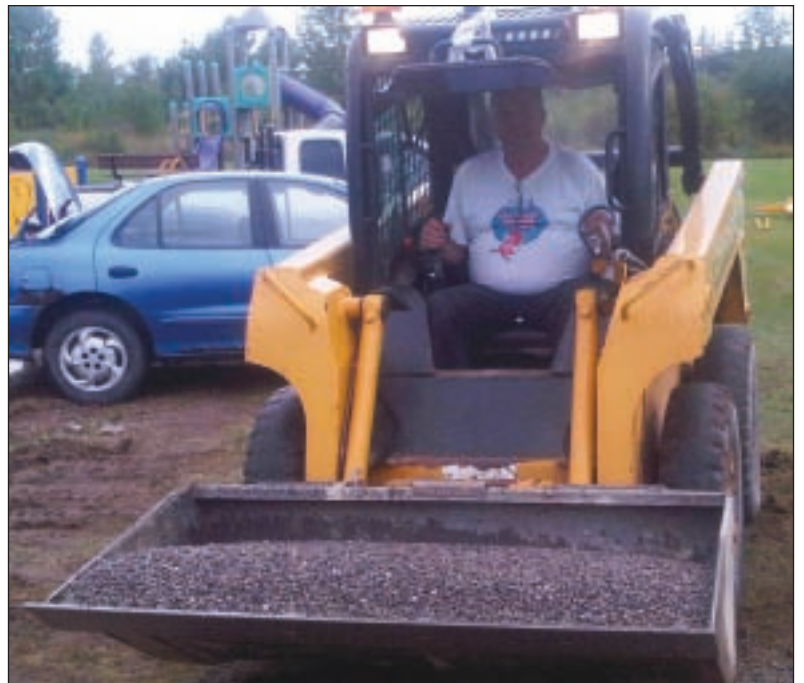
Mayor Hec Helping on Build Day
